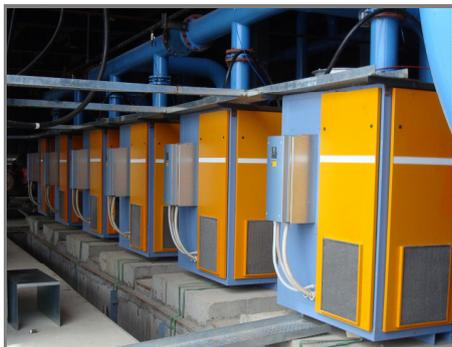
The systematic replacement of water cooled pumps with Pneumofore UV50 units at HNG involved in 2012 the Naidupeta and Nashik plants, where a new logic was installed, combined with a Variable Speed drive and an Ethernet card for each vacuum pump.
