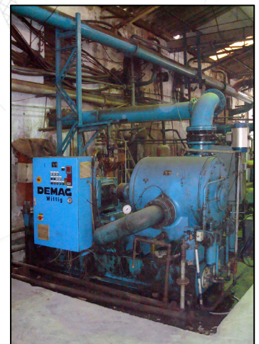
Replaced Wittig WPSO Pumps
