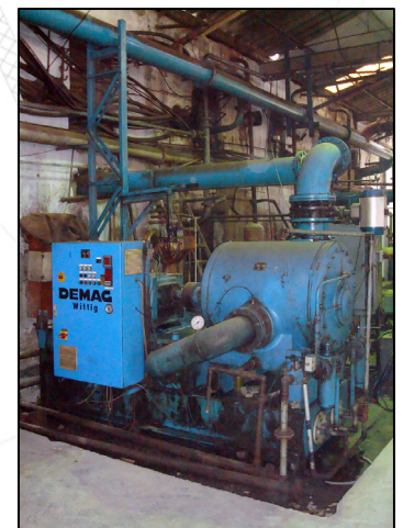
Replaced Wittig WPSO Pumps
