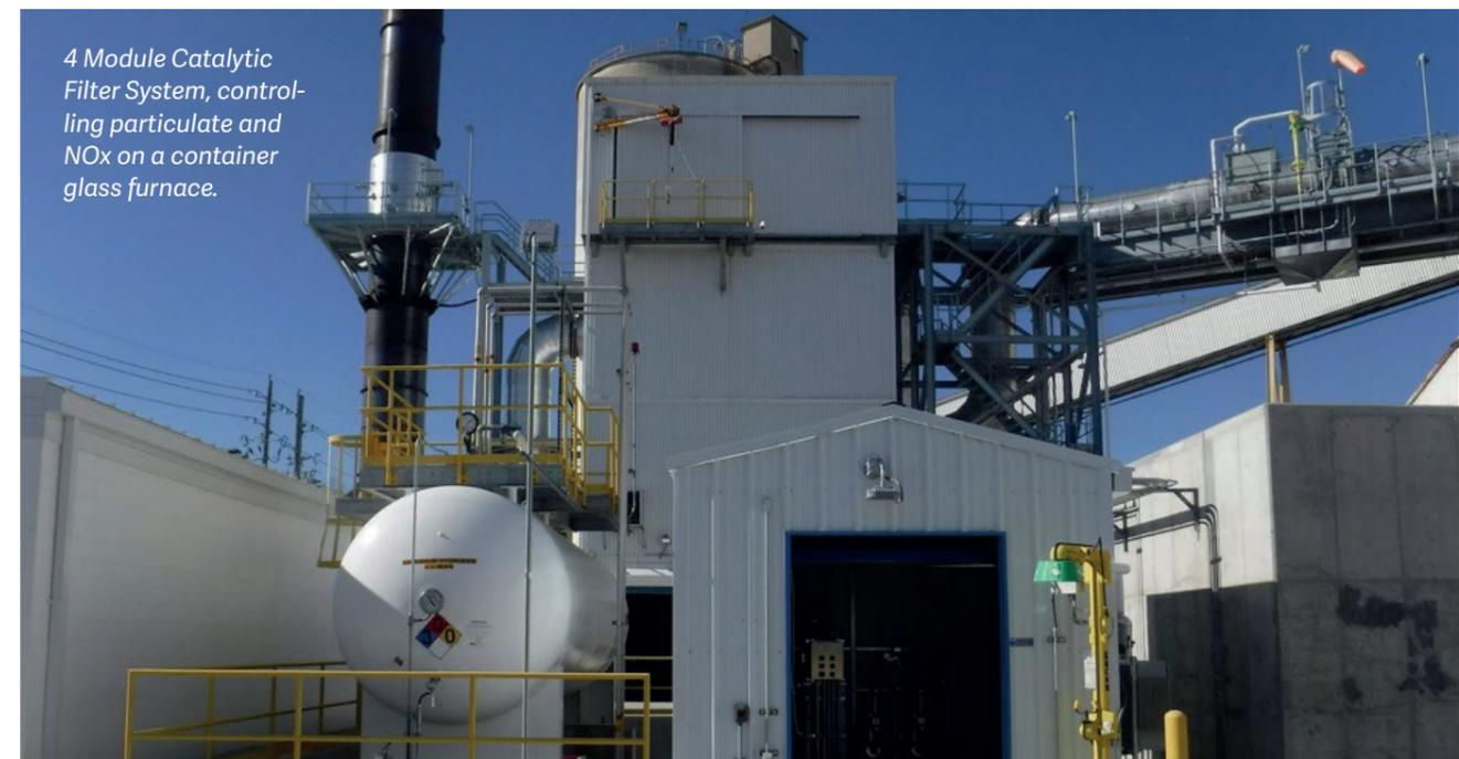
4 Module Catalytic Filter System, controlling particulate and NOx on a container glass furnace.
