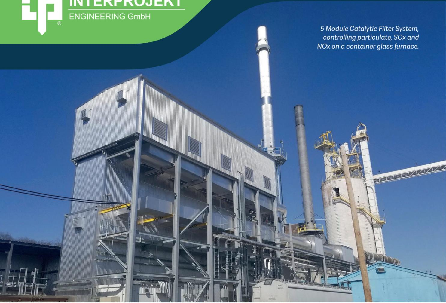
5 Module Catalytic Filter System, controlling particulate, SOx and NOx on a container glass furnace.
