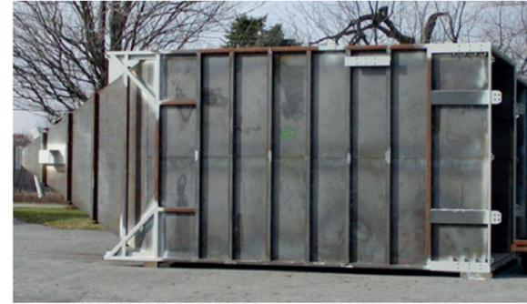
A catalytic filter module delivered to the jobsite and ready to be rigged for lifting.
