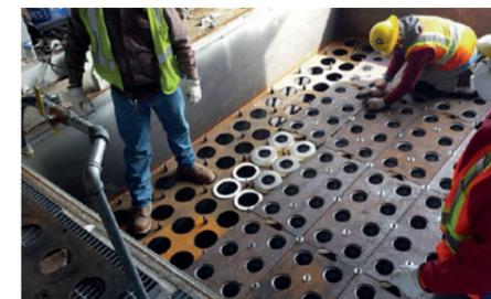
*With the top lid removed, filter maintenance can be performed in a safe, ambient air environment.*
