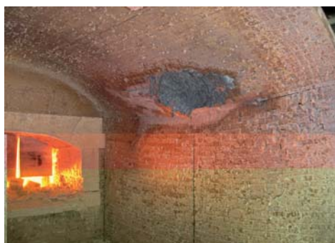
Regenerator crown after cooling down
