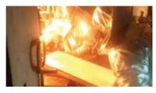
Forglass performed a hot overcoating of a flat glass furnace based in Europe.
